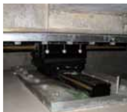
An example of residential seismic isolation application
