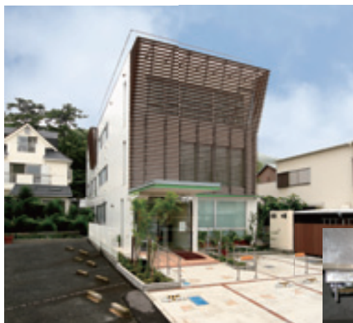
An example of residential seismic isolation application
