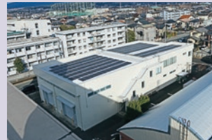
Mishima Plant THK INTECHS CO., LTD. Solar power generation
