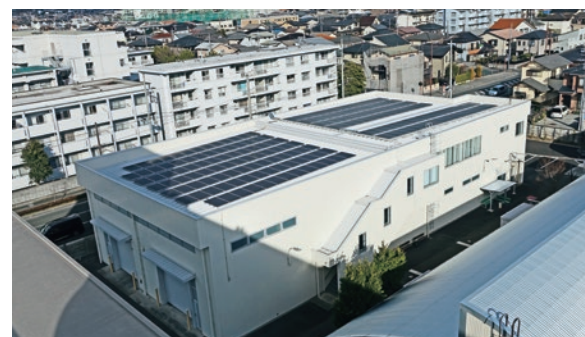
Solar panels installed on top of the development building
