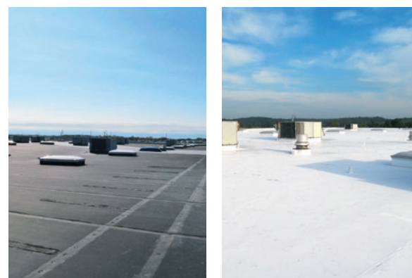
Link Ball roof before the improvement
