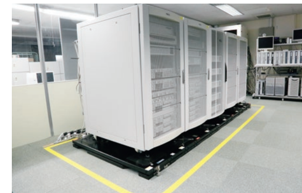
Servers that kept functioning during the Kumamoto Earthquakes thanks to seismic isolation systems
