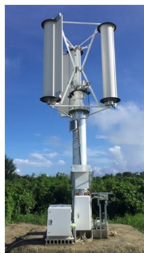
Magnus Vertical-Axis Wind Turbine set up in Nanjo, Okinawa Prefecture
