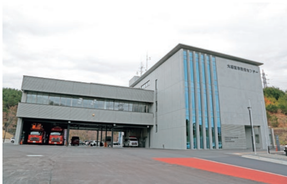
Front view of the Ofunato City Disaster Prevention Center
