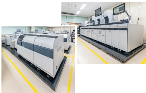
Blood analyzers (top right) and biochemistry auto analyzers (bottom left) installed with seismic isolation systems
