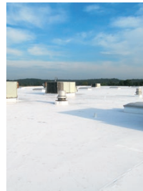
Roof after the improvement
