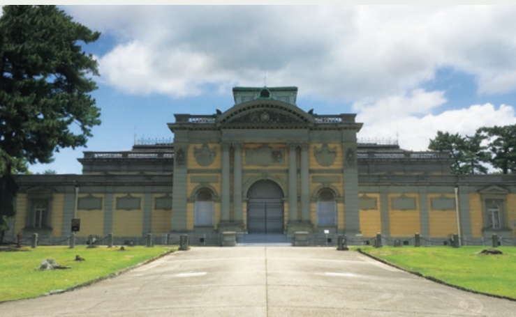
Western facade of the Nara Buddhist Sculpture Hall (Former Imperial Nara Museum Original Museum Building), designed in a Western style
