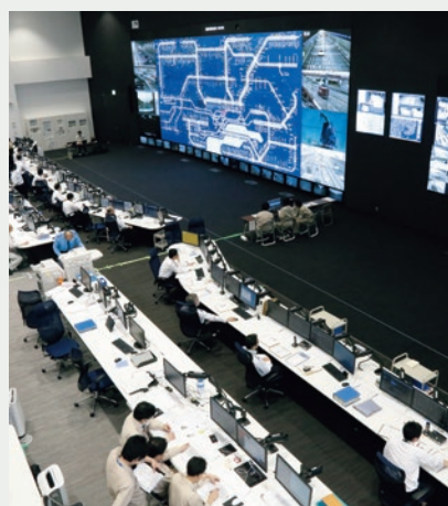
Control room with seismic isolation devices in the floor
