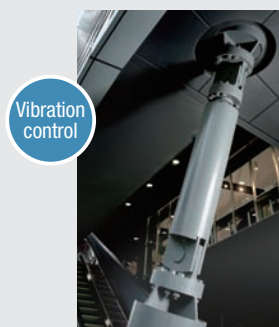
RDT viscous damping system used for vibration control
