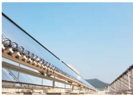
Solar power is collected to heat the plant's water. Some of the water is used for the plant's showers and heating system.
