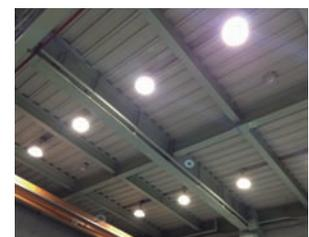
At THK Manufacturing of Europe, 260 mercury lights inside Factory 1 have been replaced with LED lights, reducing annual energy use by 40,000 kilowatt-hours. This has also improved visibility by increasing the average brightness measured at 45 locations within the factory from 231 to 368 lumens. The lights in Factory 2 are scheduled to be converted to LED in 2015.
