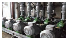
Coolant pump motors.
