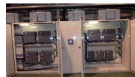
Inverter control panels.
