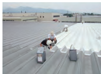
Coating the roof. The white substance is an anticorrosive base coat.
