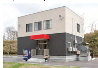
Equipped with seismic isolation, solar panels, rainwater tanks, and provisions needed for business continuity, the new building houses Myotoku's server computers.
