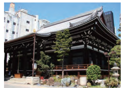
Honnoji: Seismic damping has been provided under the floor and roof, and seismic isolation tables support the statuary in the main hall.
