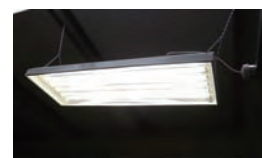
Energy-efficient lighting at TMI.
