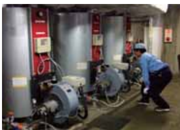
Periodic boiler inspection
