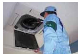
Inspecting air conditioner filters in the assembly bay
