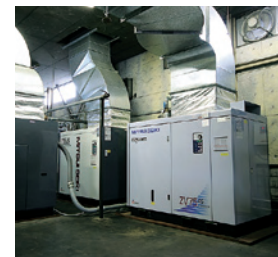
Inverter-controlled air compressor installed at the KOFU Plant
