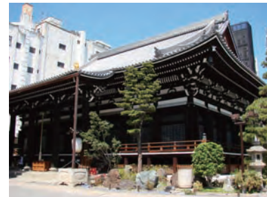
Honnoji: Seismic damping has been provided under the floor and roof, and seismic isolation tables support the statuary in the main hall.
